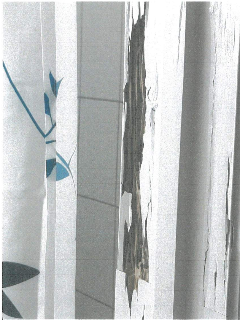
Bathroom door frame damaged by termites.
